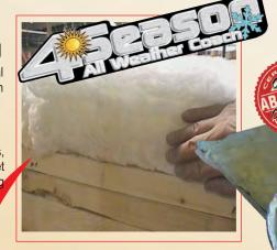
insulation and the tank itself is wrapped with an Astro-Foil blanket.
