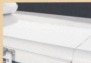
1-YEAR OLD ITASCA FIBERGLASS ROOF
