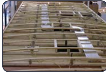
5" Roof Truss with Ducted AC and Walkable Decking
