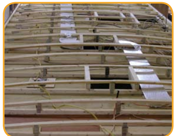
5" ROOF TRUSS WITH DUCTED AC AND WALKABLE DECKING
