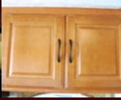
Raised Panel Cabinetry
