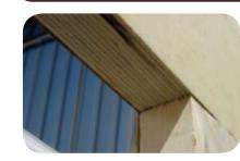
Micro-lam (laminated wood headers) are used in slideroom openings. These eliminate the warping that many other manufacturers experience.
