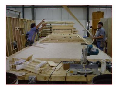
Sidewalls and partition walls are built on jigs in order to maintain uniformity. Paneling is glued & mechanically fastened. The walls are then set, & attached to the unit, and cabinetry is prepared for installation. The walkable roof is made with 3/8" O.S.B.
