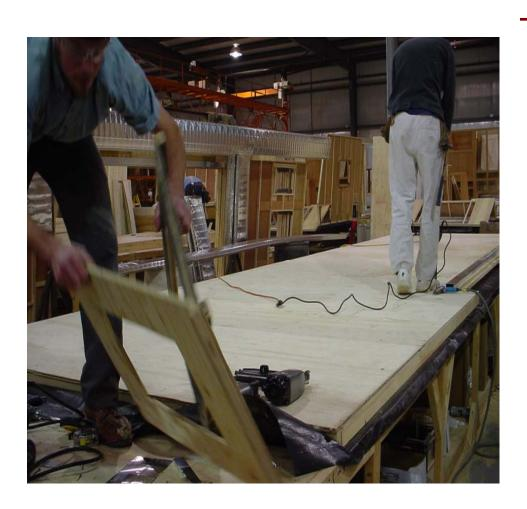
The floor is built in a jig using 2X3 floor joists placed 16" on center. It is insulated using R-7 fiberglass. Heat ducts, plumbing & wiring are then installed & the belly is wrapped with Darco<sup>™</sup> to protect it from the elements. It is then sheathed with 5/8" tongue & groove plywood.
