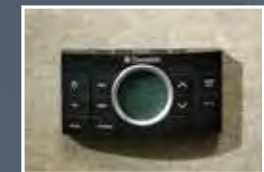
Dual zone thermostat for living room and bedroom A/C
