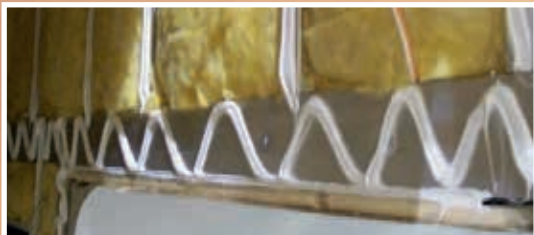
Thick Silaprene (475 PSI) guarantees solid contact between the gelcoat and aluminum frame without lamination
