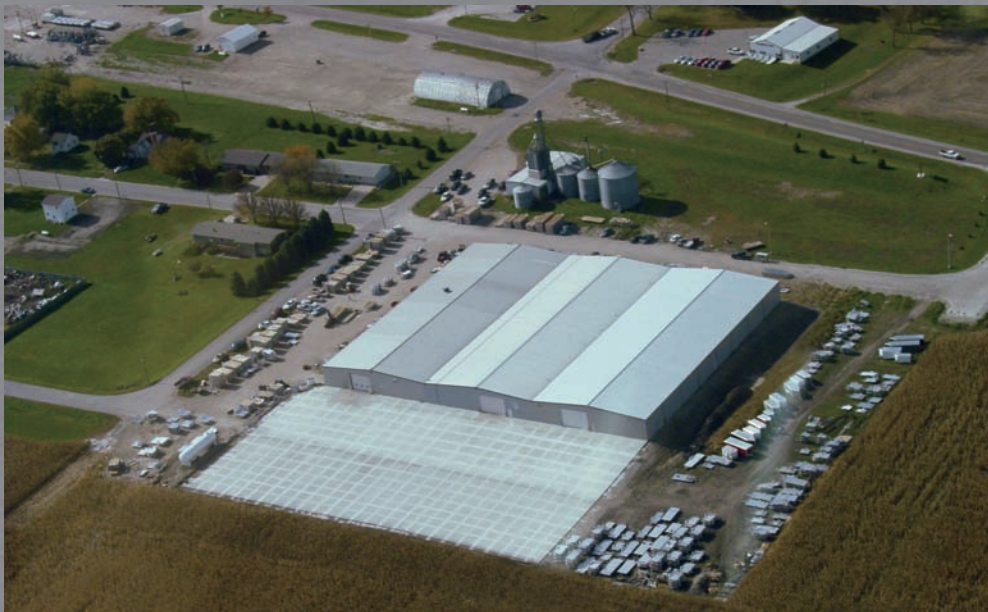
Aerial view of Aluma factory
