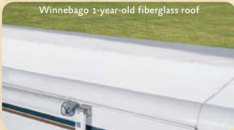
Winnebago 1-year-old fiberglass roof
