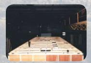
Springdale utilizes crowned, residentialstyle, 41/2" truss rafters, shown here with air conditioning channels to accommodate our ducted roof/air option.
