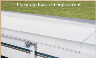
1-year-old Itasca fiberglass roof
