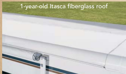
1-year-old Itasca fiberglass roof
