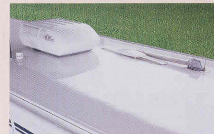
One-year-old Winnebago Industries fiberglass roof
